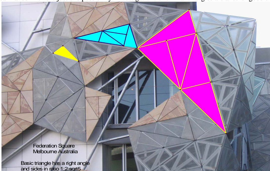
Figure 3 Federation Square, Melbourne, showing how the pattern is constructed from tessellating triangles.
